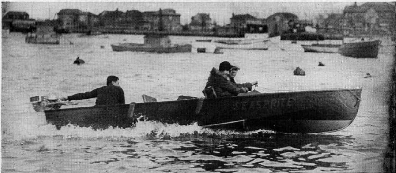
With from 16 H.P. to 22 H.P. this 16 ft. Baby Buzz travels twenty to twenty-seven miles
